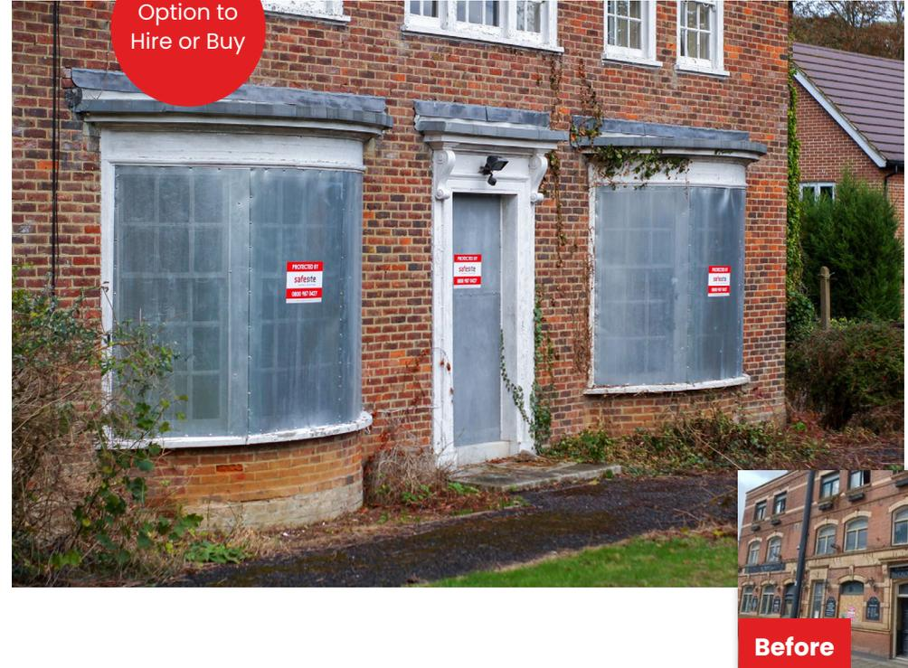
Our expertly installed tamper proof galvanised and perforated steel security screens provide vacant sites cost-effective protection from squatters, vandals and thieves, while allowing natural light to enter. Ideal for a variety of premises, vacant property security, occupied property security, storage, warehousing, temporary works security.
